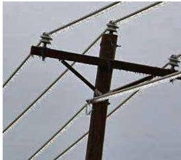
ice on top of the lines to near three quarters of inch on top. These are not circumference figures, but ice accumulations from the top of the line to the top of the ice. Below the lines the ice accumulation was even thicker.
