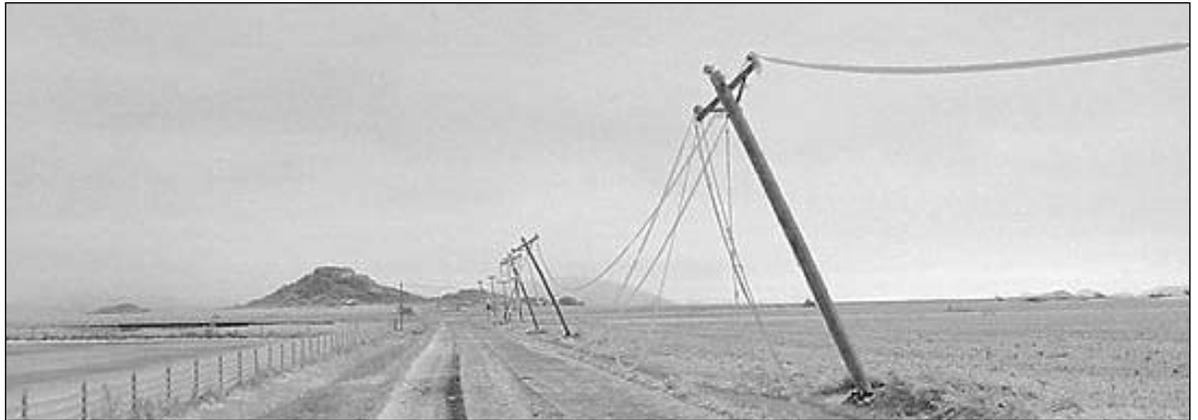
*Kiwash Electric power lines buckle under the heavy weight of ice. PHOTO/LISA WILLARD.*
